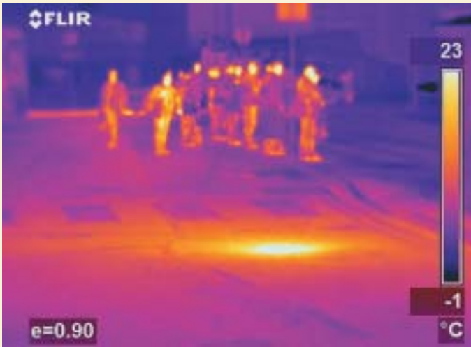
The leak in the pipeline can be clearly located thanks to infrared.
